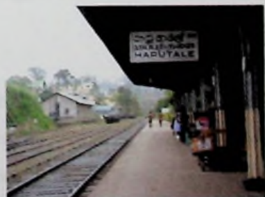
Fig:1.19 Railway station Haputale. Source:Ranga.
