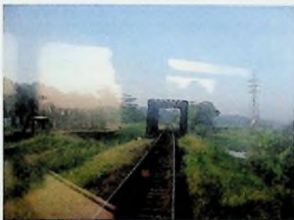
Figure. 1.15 Recent constructions of railway bridges at Colombo suburbs Source: Ranga
