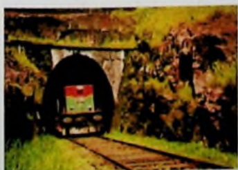
Fig. No.1.14 Tunnel No. 41 at Demodara. Source- Ranga
