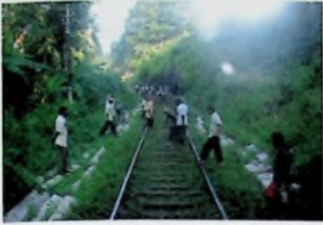
Figure.1.16 Maintenance of railway tracks Source : Ranga
