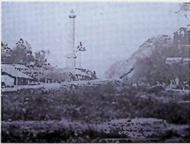
Fig. No.1.8 Captain Doston Pillar. Source: History of Railway Transport.
