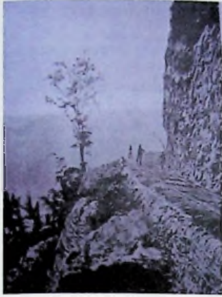
Fig.No: 2.13 Kadugannawa Pass Source: History of railway transport
