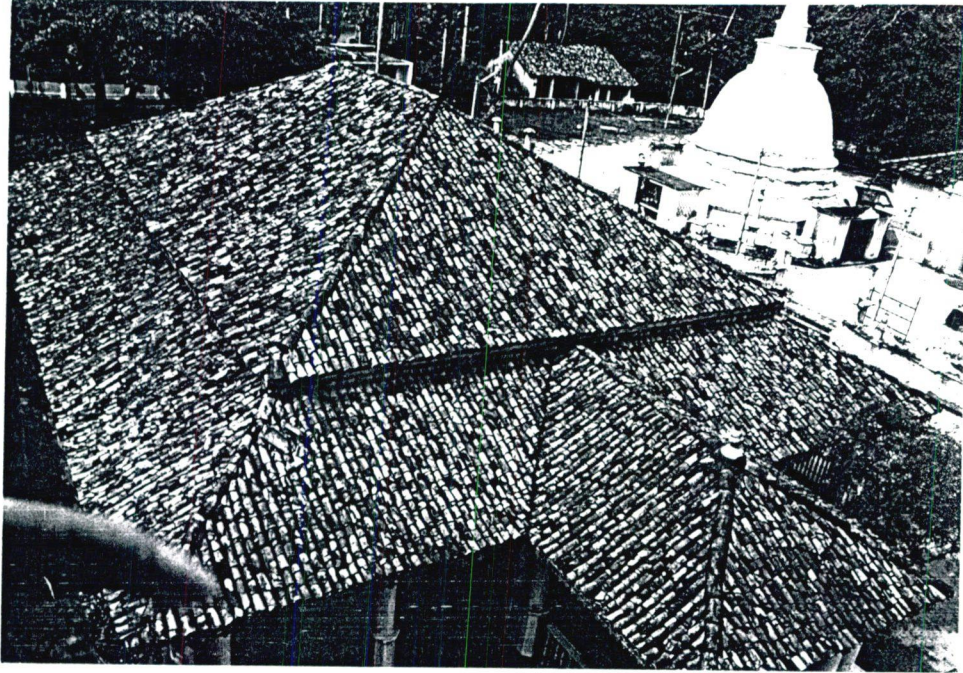
Fig 115 Double hip roof -Sunandarama viharaya
