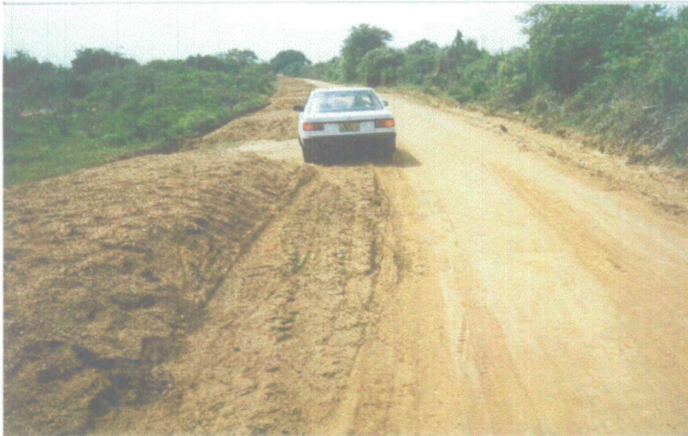
Figure 8.3 Stagnation of water due to the gravel piling
