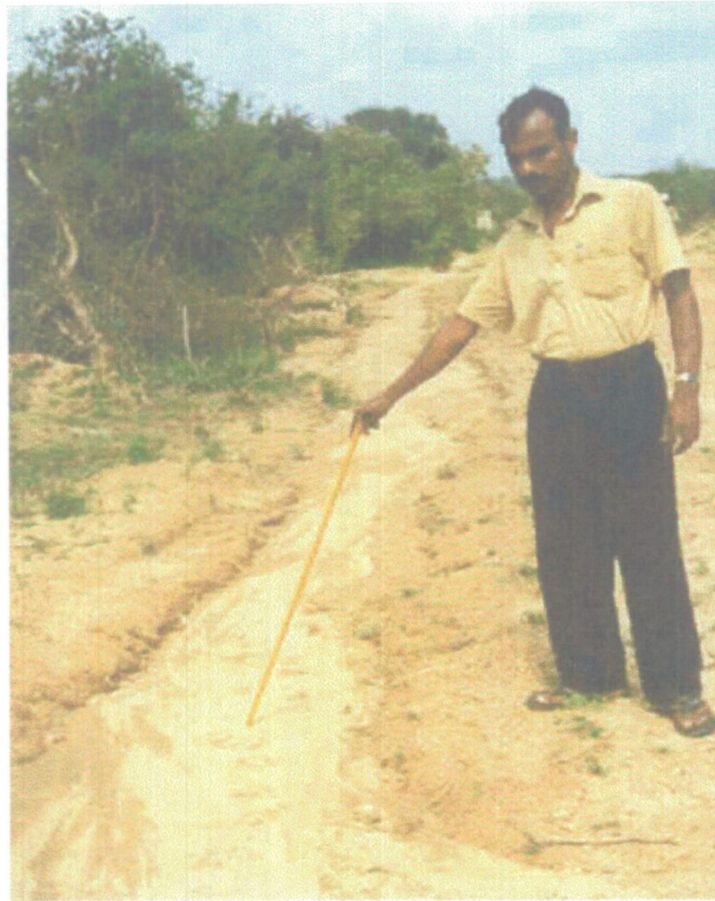
Figure 8.5 Siltation of drains.
